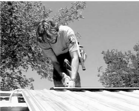
Casa Verde Builders YouthBuild installing an aluminum roof
