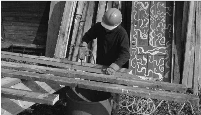
ReCycle North of Burlington, Vermont, deconstructs old buildings; up to 80 percent of the resultant materials can be reused.
