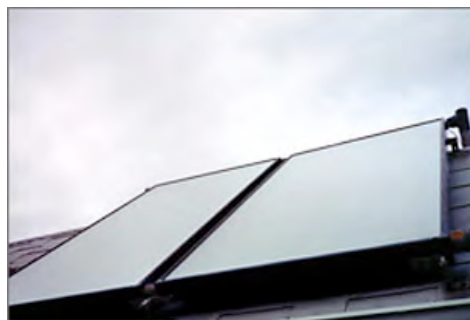
For solar hot water systems, flat-plate solar collectors are typically installed facing south on a rooftop. Photo courtesy of www.nrel.gov .
