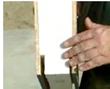
Structural Insulated Panel section. Courtesy of www.consumerenergycenter.org
