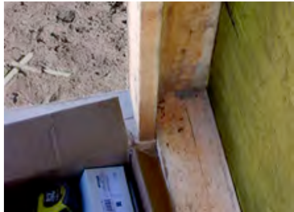
Two-stud corner framing. Used with permission of the Nebraska Energy Office
