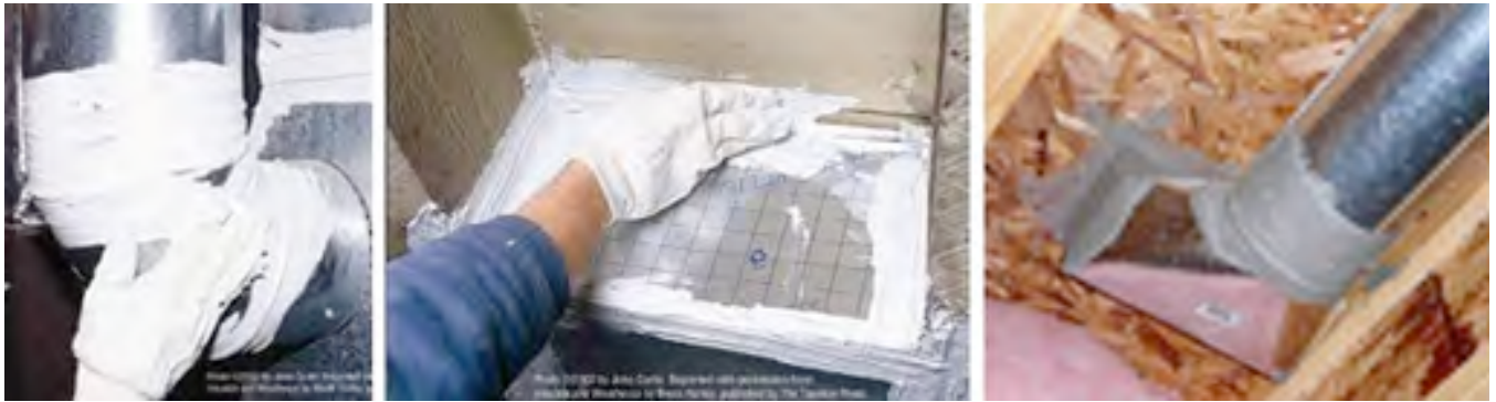
Duct connections should be sealed with mastic-hardcast or UL181 foil tape, not duct tape.
