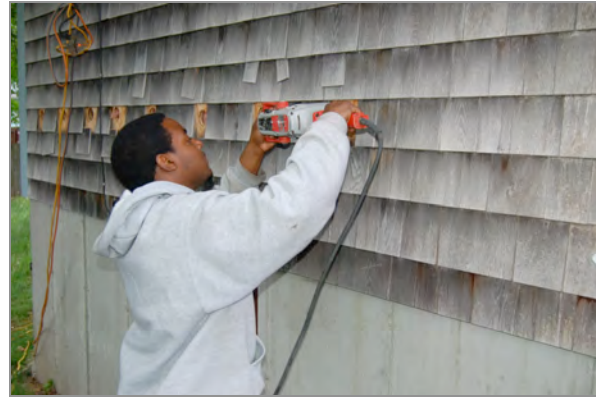
Holes are drilled into the exterior to blow insulation into the walls.
