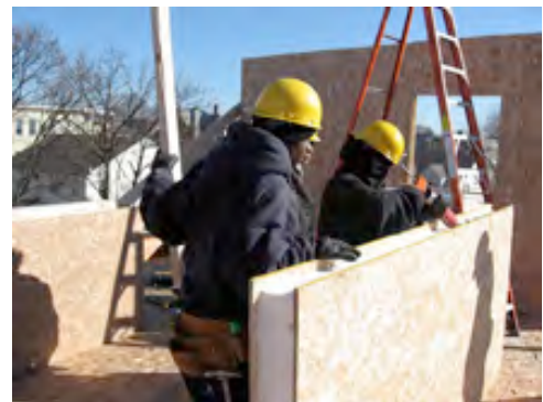
Structural Insulation Panels (SIPs) Source: Energy Star Thermal Bypass Checklist
